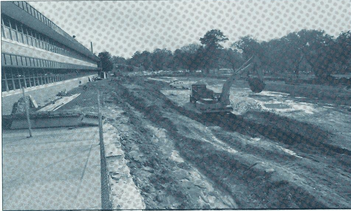
Ground Breaking at the Bobby E. Leach Student Recreation Center
