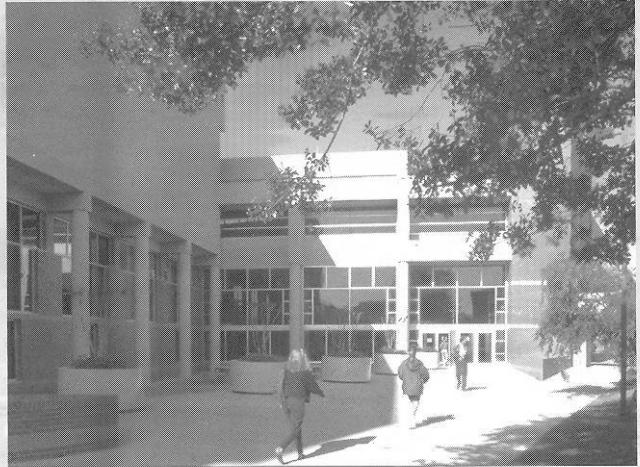
The Dr. Bobby E. Leach Center, a state-of-the-art student recreation facility, with an indoor pool, saunas, basketball and racquet-sport courts, was completed in 1991. And in June, a 2300 square foot free weight area was completed.
