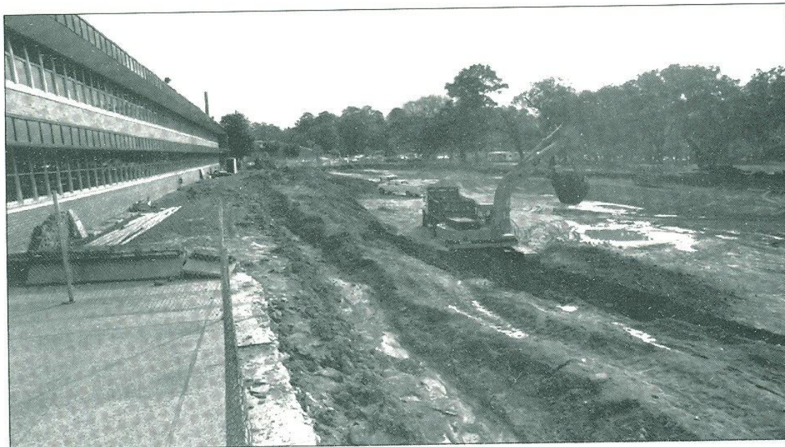
Ground Breaking at the Bobby E. Leach Student Recreation Center
