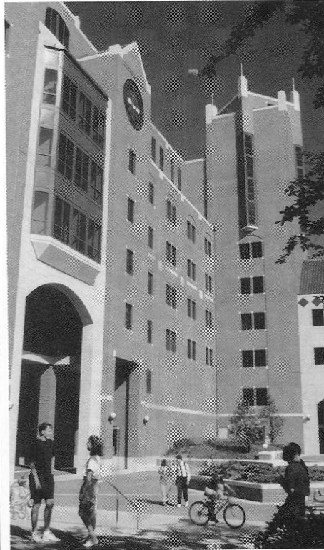
The University Center is one of the most popular buildings on the FSU campus.
